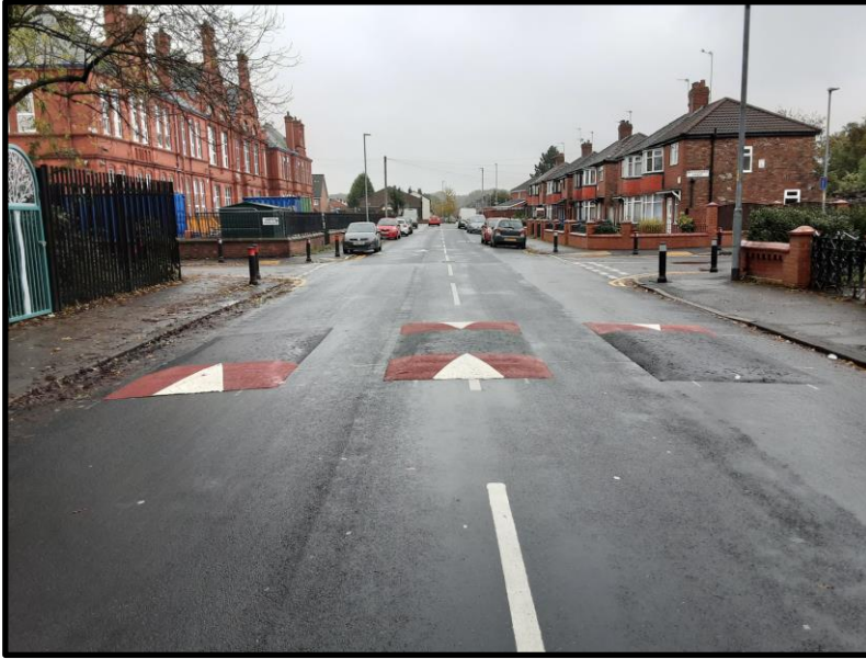
Lily Lane/Lizmar Terrace, Moston - Raised junction/speed cushions/crossing points/kerb build outs/bollards/No Waiting at any time restrictions
